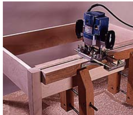
9--Clamp scrap to the rear apron to provide a base for the router, then cut the hinge rabbet using a straight bit.
